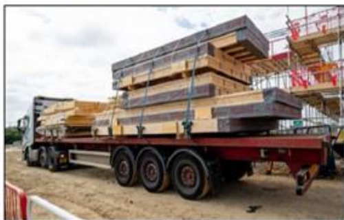
7 – Delivery to site
